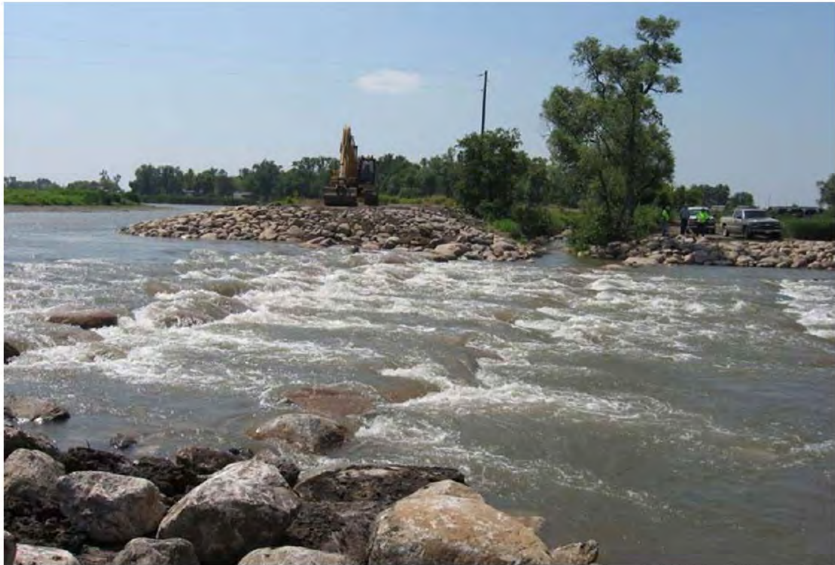
Figure 91. Rapids replacing dam to provide grade control and facilitate fish and canoe passage. Reconnecting Rivers: Natural Channel Design in Dam Removals and Fish Passage , p. 80. Minnesota Department of Natural Resources Ecological Resources Division, 2010.
